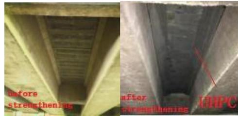
Fig.3 the effect drawing of UHPC
